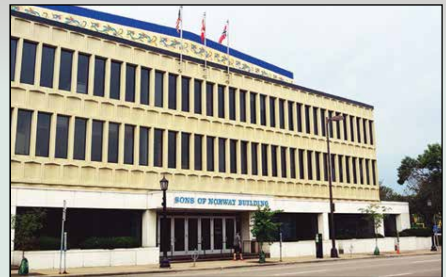
Demolished Sons of Norway Headquarters, located in Minneapolis, Minnesota.
