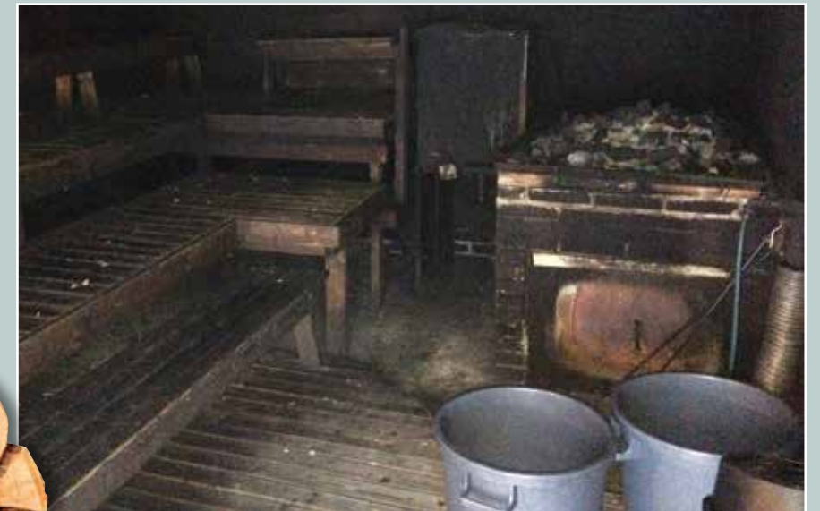
Old style “smoke sauna” had no ventilation, and walls were blackened from the soot and smoke from the fire that kept the sauna hot.
