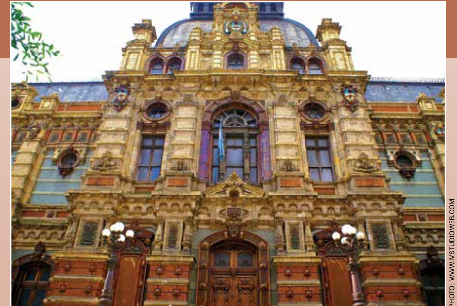
Ornate main entrance of the Water Company Palace—(Aguas Corrientes Palace).
