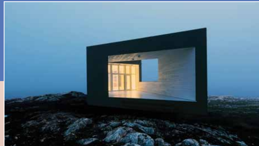
Fogo Island Arts Colony structure.
